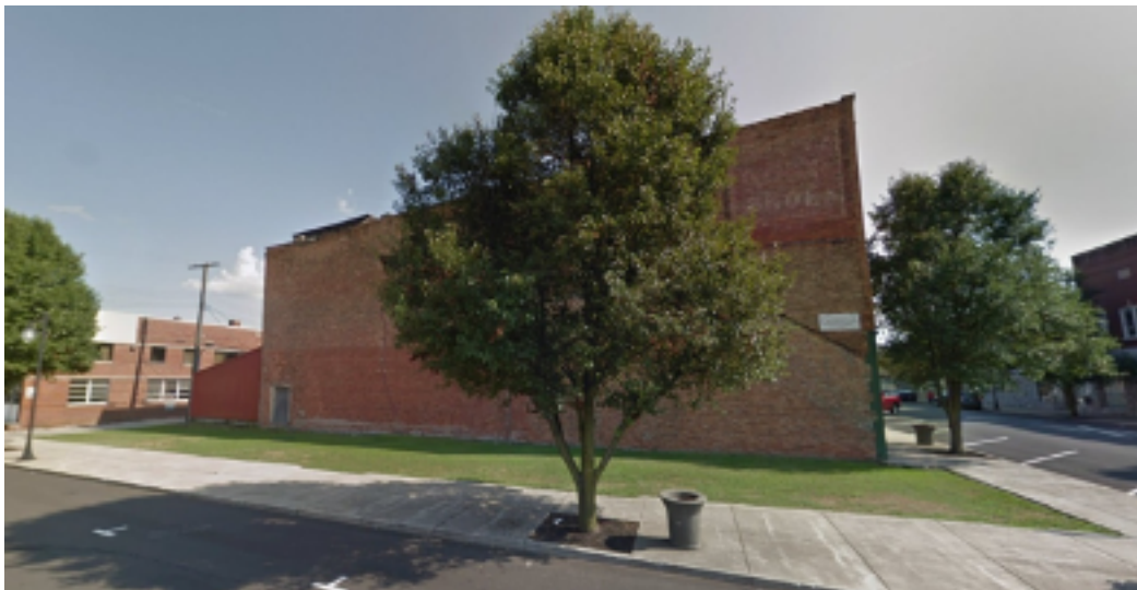
Figure 58: Existing conditions of the pocket park.
