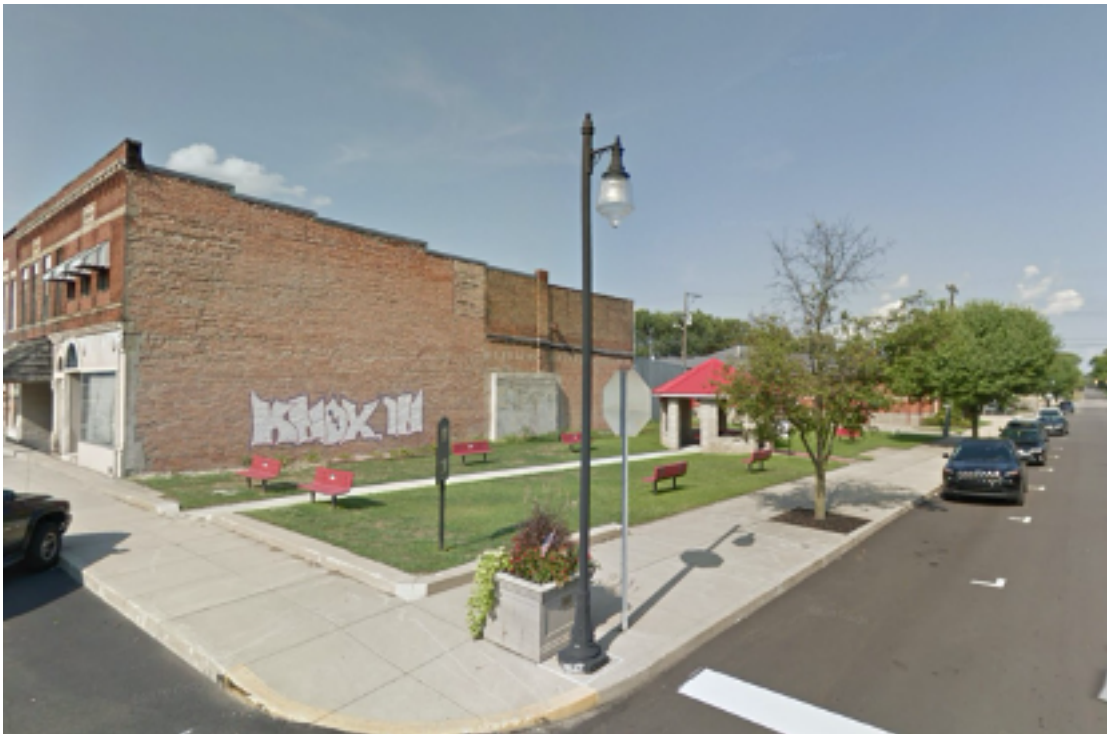
Figure 56: Existing conditions at Serenity Park.
